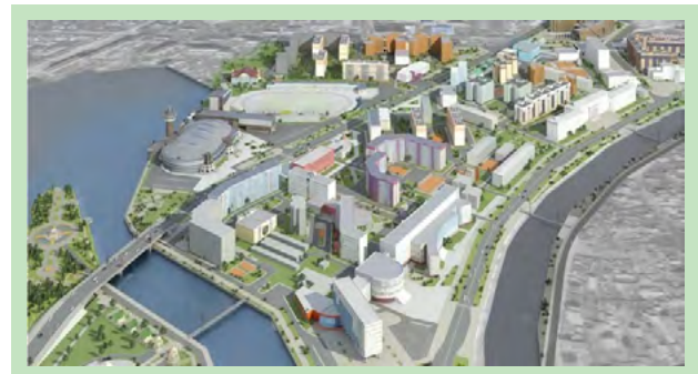
The main campus of the North-Eastern Federal University in Yakutsk. (Photograph courtesy of NEFU)
