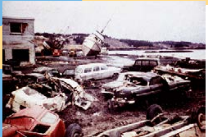
Close-up of tsunami damage along the waterfront at Kodiak. (Photograph courtesy of USGS)
