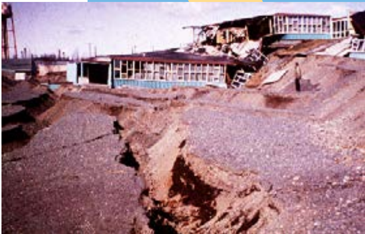
Part of the bluff on which Government Hill Elementary School in Anchorage was built slid southwards 35 feet. (Photograph courtesy of USGS)
