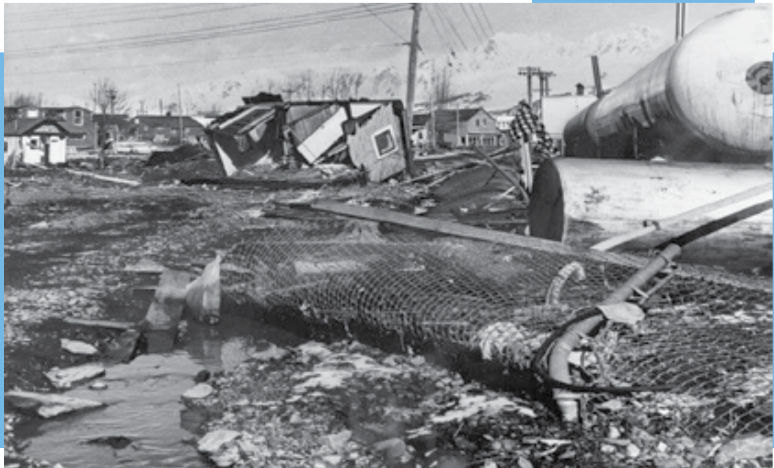
Damage to the town of Seward after quake and tsunami. (Photograph courtesy of Wikimedia Commons)
