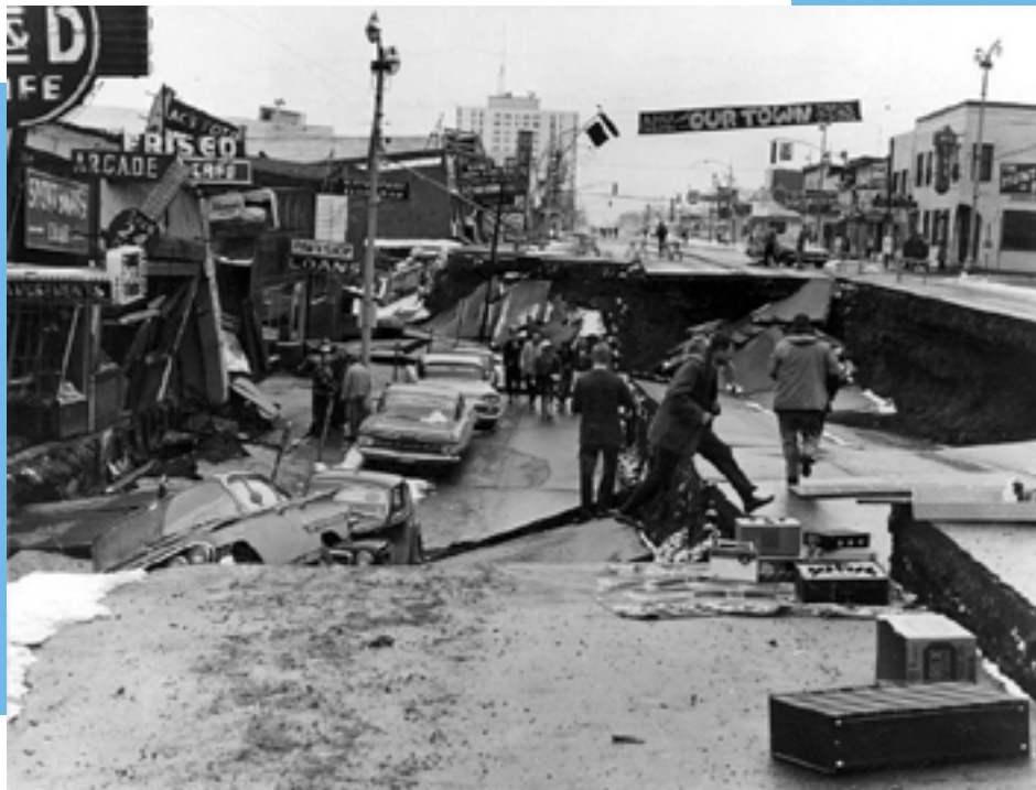
Iconic image of damage to Fourth Avenue, downtown Anchorage. Before the earthquake, the sidewalk at left, which is in the trough, or graben, was at street level on the right. The graben subsided 11 feet in response to 14 feet of horizontal movement. (Photograph by Joseph K. McGregor and Carl Abston, courtesy of USGS)
